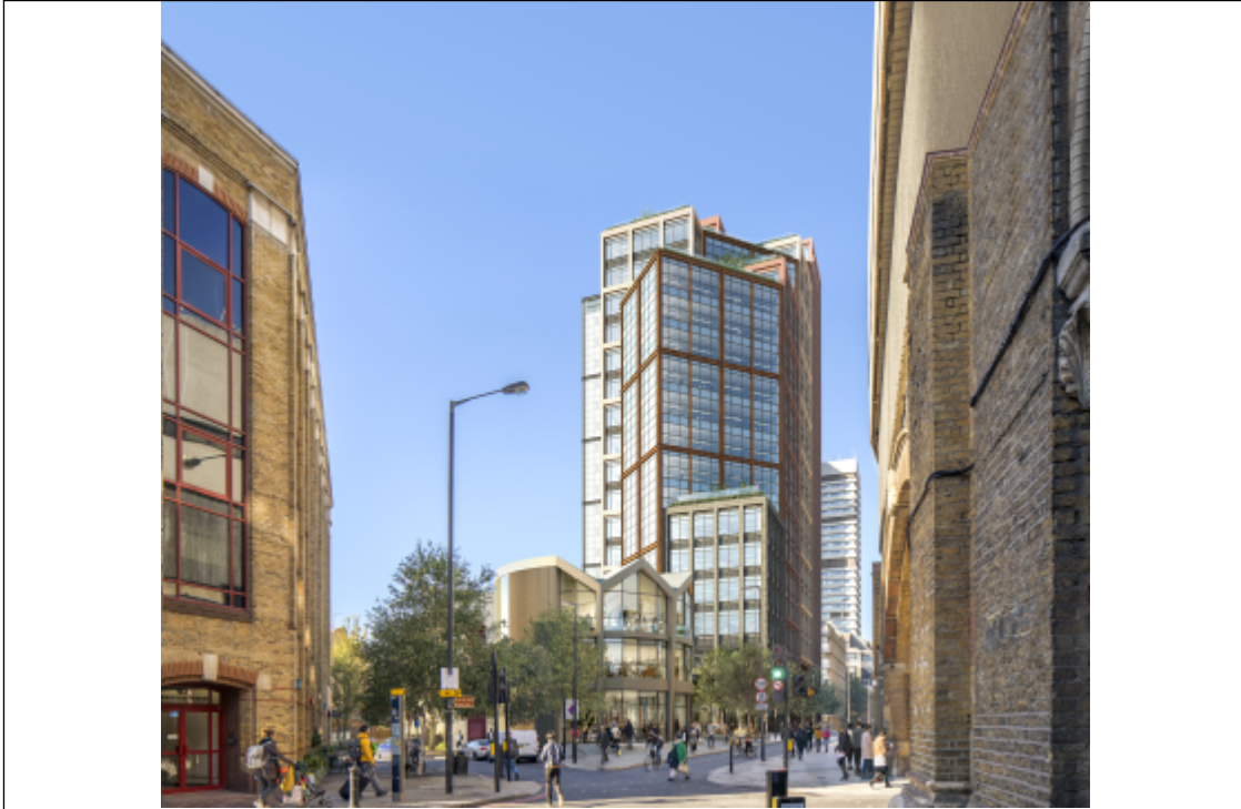
Image – View along St Thomas Street
