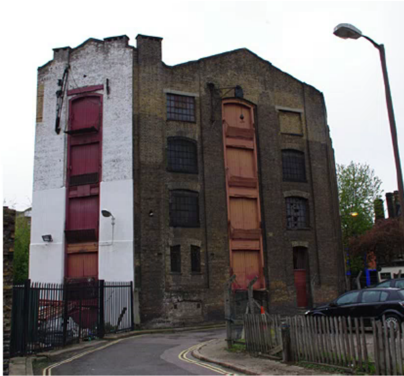
View of East and North Elevation of the Vinegar Yard Warehouse
